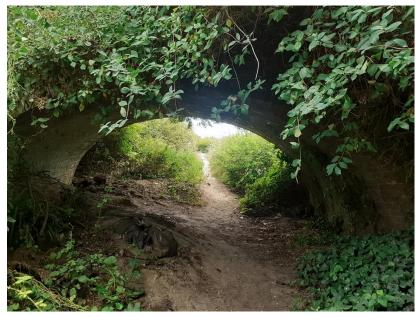
Burndell Bridge is not in the best condition. The bridge is heavily overgrown and only the underside of the arch and parts of the approach walls visible. Once are the undergrowth has been cleared a better assessment of the work to be undertaken can be made. It is believed that any distortion and cracking of the bricks can be overcome by careful repair without the need for rebuilding. The wing walls are cracked and pushed
