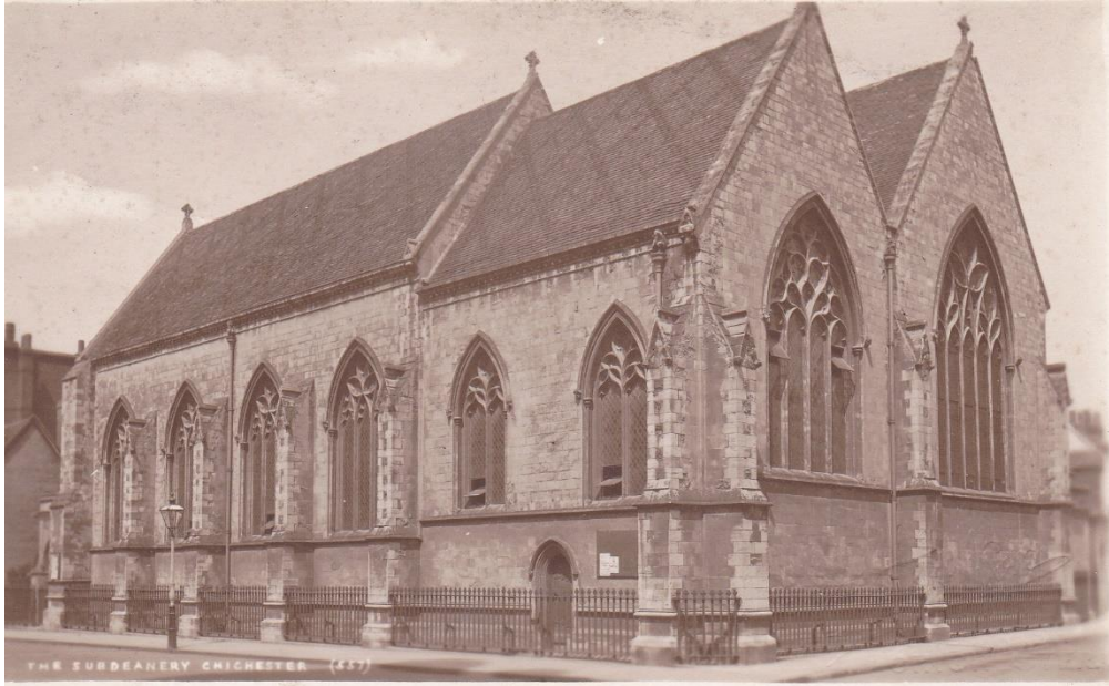
The Church of St Peter the Great in West Street, built 1848-1852 to a design by R C Carpenter to rehouse the St Peter's congregation from the Cathedral. At the time of this tale – 1851 - the incomplete church had been licensed for use but had not been consecrated. (Author's collection)
