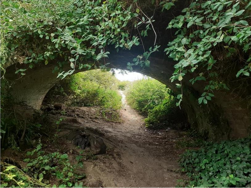
Burndell Bridge is not in the best condition. The bridge is heavily overgrown and only the underside of the arch and parts of the approach walls are visible. Once the undergrowth has been cleared a better assessment of the work to be undertaken can be made. It is believed that any distortion and cracking of the bricks can be overcome by careful repair without the need for rebuilding. The wing walls are cracked and pushed
